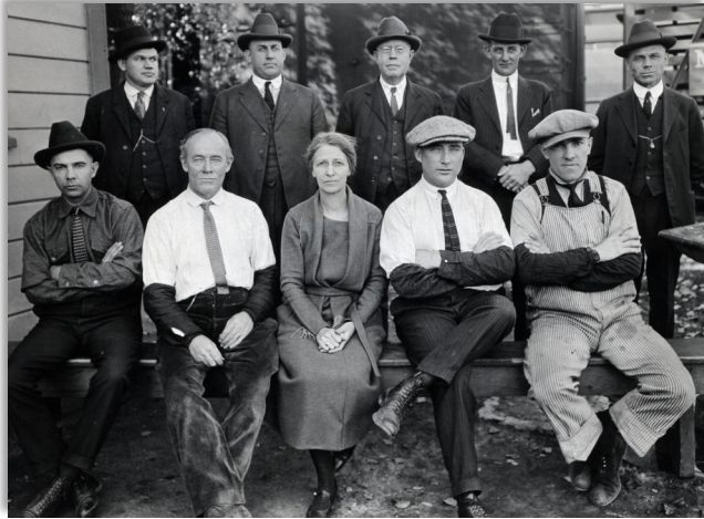
SP Yard Office Staff @ Roseville
